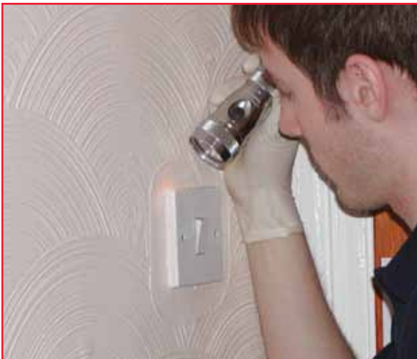
• Remove and inspect light switch covers
